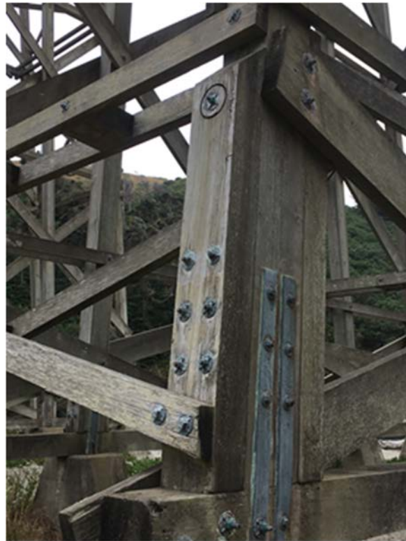
Figure 3: Bolstered exterior columns
