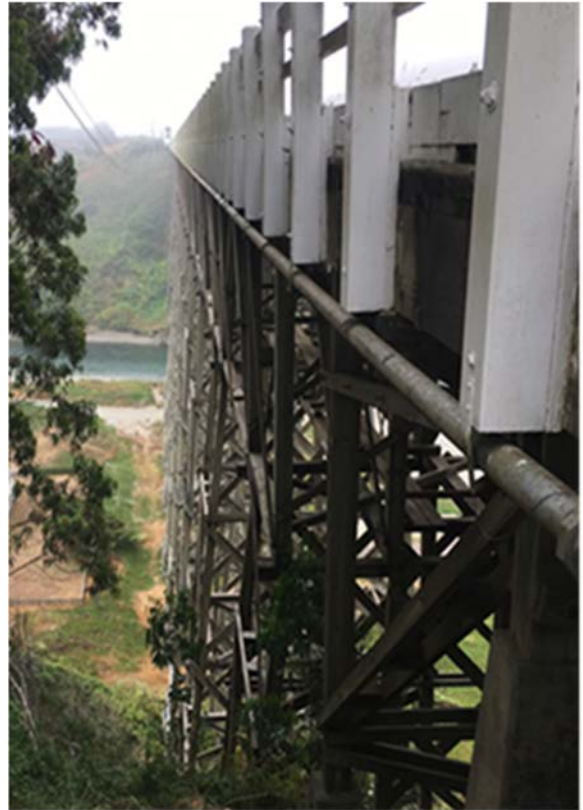
Figure 2: Good dimensional integrity of trestles
