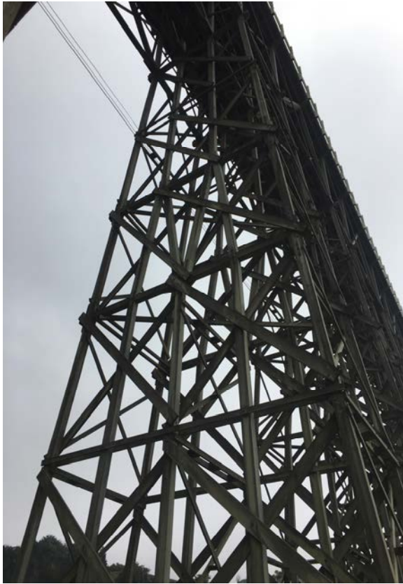
Figure 1: Battered columns provide wide base below roadway
